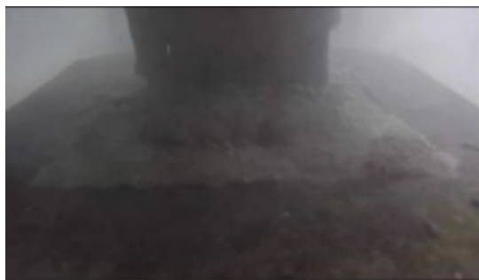
Figure 6 Casting mortar under water
