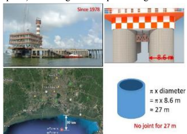
Figure 1 Structure to be repaired and its site location at Samut Prakan
